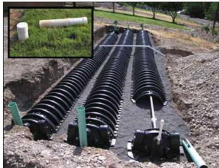
This conventional port has several drawbacks. First, the homeowner is faced with the six curious ports sticking up in the lawn when the job is done. The slip caps are hard to remove, and that often results in the entire port being extracted from the ground instead of just the cap (inset photo).
