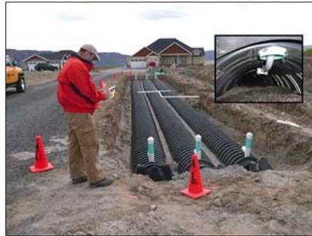
The inset photo shows the underside of the port inside the vault with the lateral end sweep turning up into the port body. The end orifices in each lateral point down into an orifice shield to drain each lateral at the end of the dose. This is very important in colder climates where the laterals could freeze and burst.
