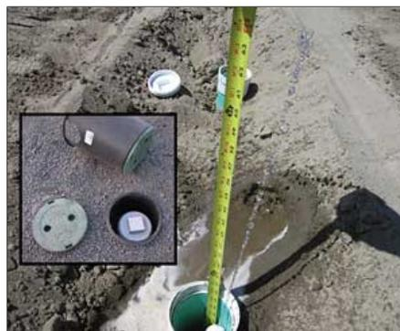
The inset photo shows the finished appearance of the drainfield port using a 7-inch round irrigation valve box, which provides plenty of space for the 4-inch port and its threaded cap.
